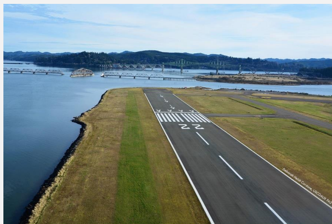
Above: Taking off from Sector North Bend with the Conde McCullough Memorial Bridge and Coos Bay Rail Link Swing Span Bridge in the background. 02JAN18
